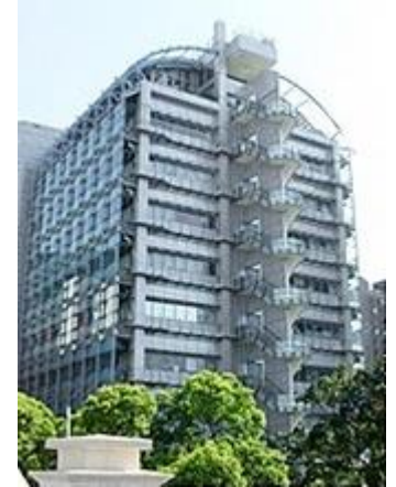
Kadoorie Biological Sciences Building
